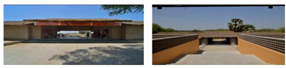
The new Centre, designed in an honorary capacity by architects, Karan Grover & Associates, is a 'Green' building made of compacted mud bricks and in keeping with the terrain, covered with thatch. Though costs kept escalating due to the quality of soil and the need for retaining walls, the help received from well-wishers, along with fund raising activities, ensured that this unique building is complete.
